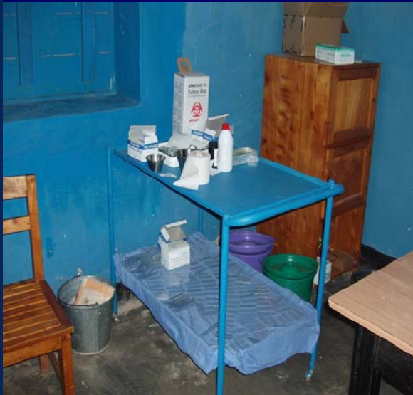
Before HIV renovation work, October 2006
